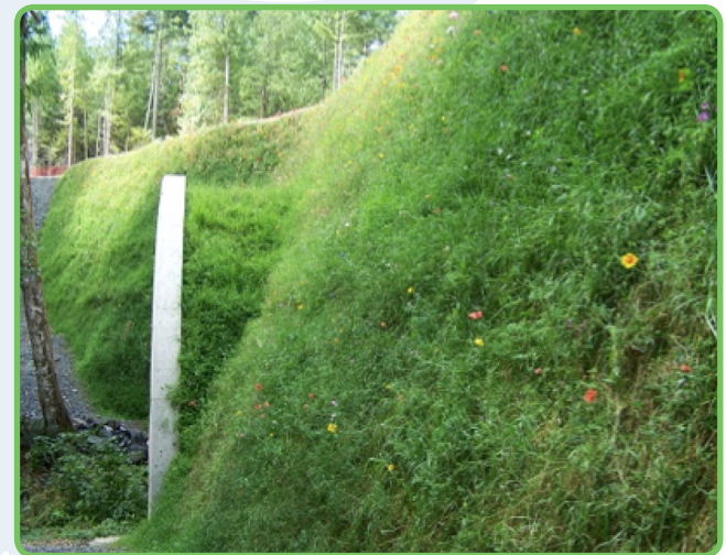
10m (33ft) tall municipal roadway
